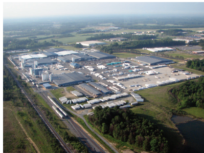
Our largest plastics plant in Monroe, North Carolina, which comprises more than one million square feet of manufacturing and warehouse space.
