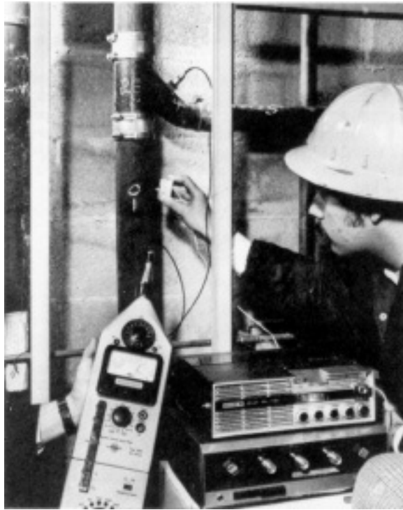
Figure 7—Testing a Hubless System.
